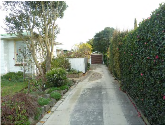
s) Liquefaction ejecta on driveway
