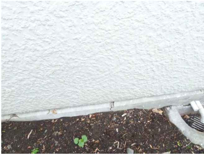
m) Foundation damage
