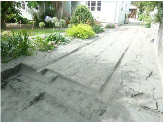
q) Liquefaction ejecta on driveway
