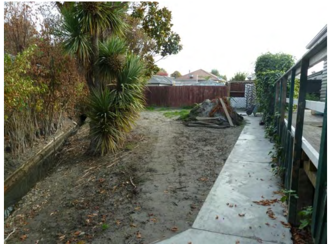
j) Liquefaction ejecta alongside culvert
