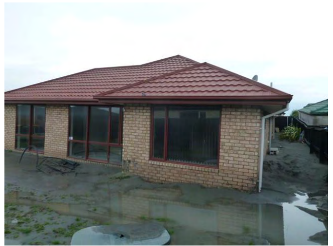
t) Large amounts of liquefaction ejecta around property
