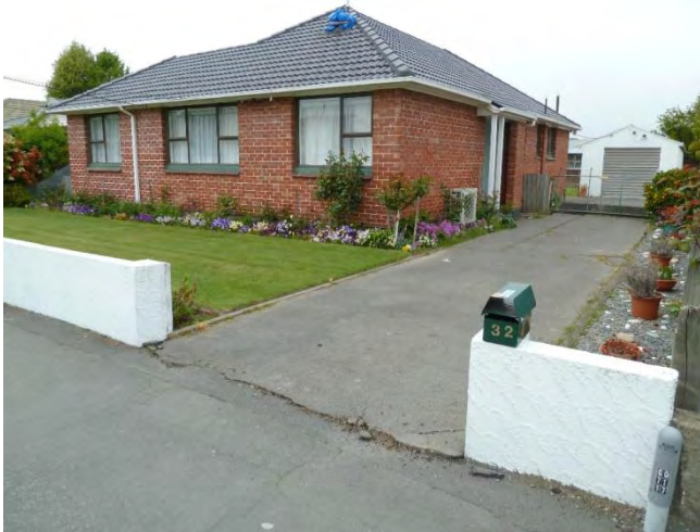
g) Damage to asphalt
