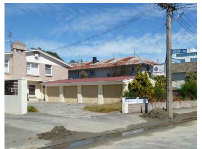
x) Piles of sand along the footpath
