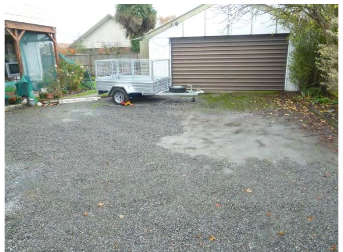
f) Isolated area of liquefaction ejecta
