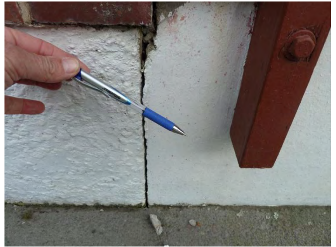
n) Foundation damage
