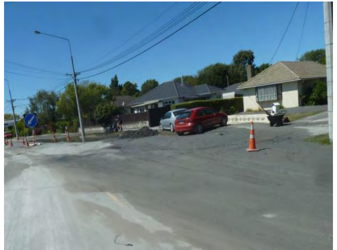
n) Liquefaction ejecta on New Brighton Road
