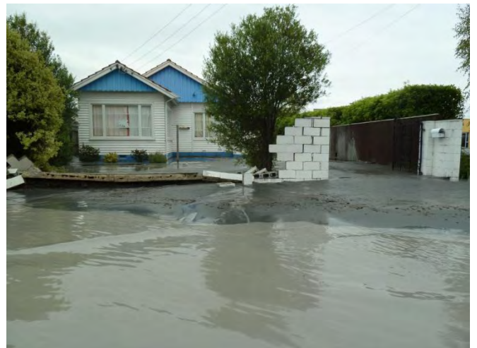
r) Liquefaction ejecta and ponding water
