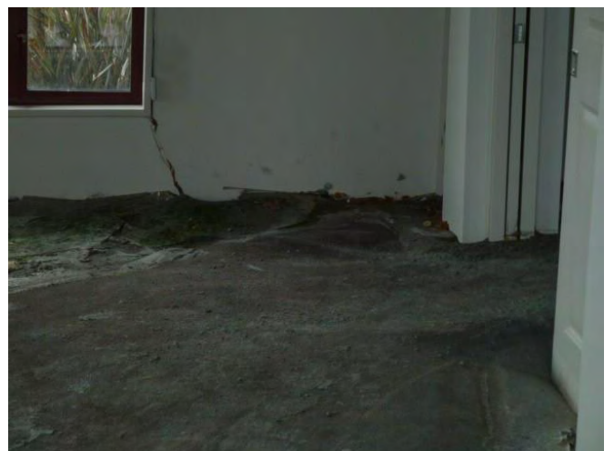
x) Large amounts of liquefaction ejecta inside dwelling
