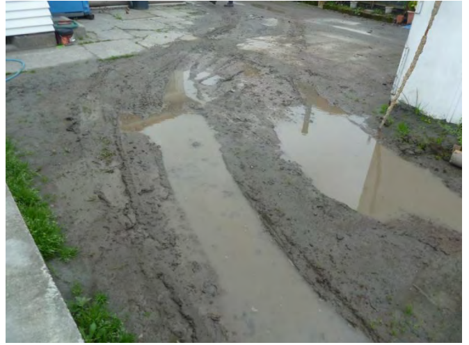
t) Liquefaction ejecta on driveway with water ponding
