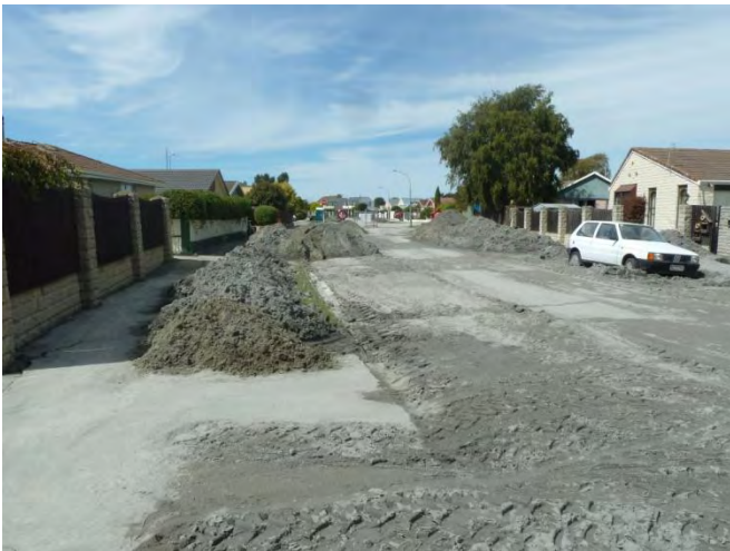
i) Liquefaction ejecta piles along Androssan Street
