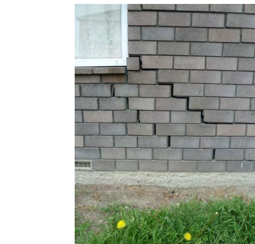
l) Brickwork damage
