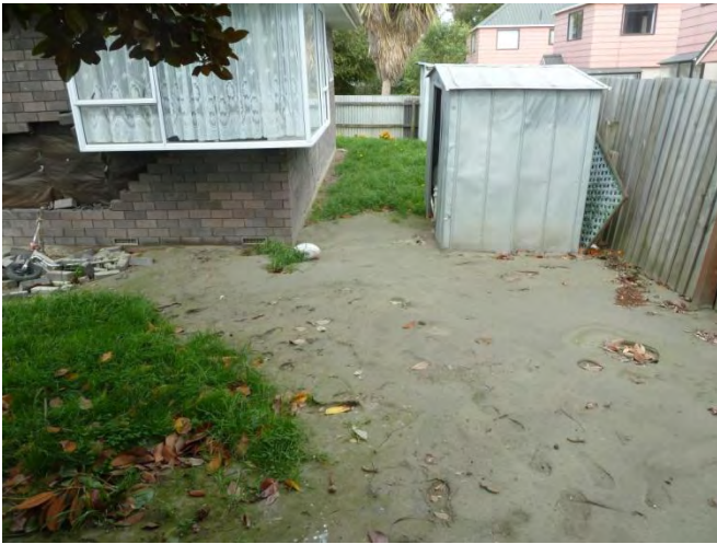
m) Liquefaction ejecta and brickwork damage
