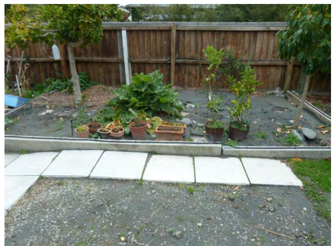
r) Liquefaction ejecta in planter with undulating pavers
