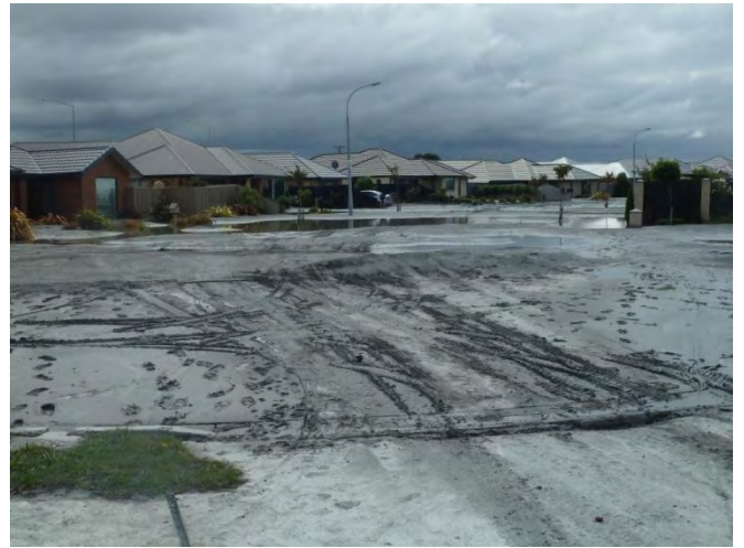
n) Liquefaction ejecta in turning circle of Seabreeze Close
