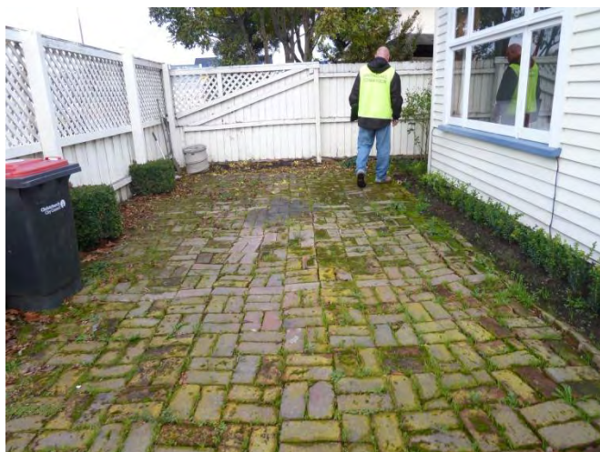
s) Undulating brick paving
