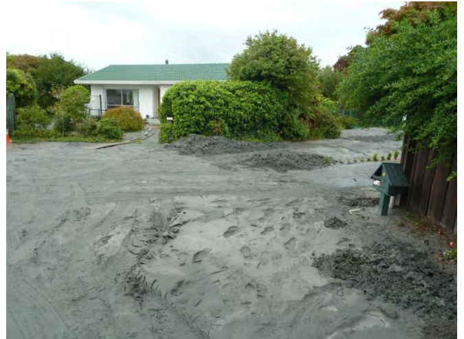
p) Liquefaction ejecta covering turning circle in Chale Lane
