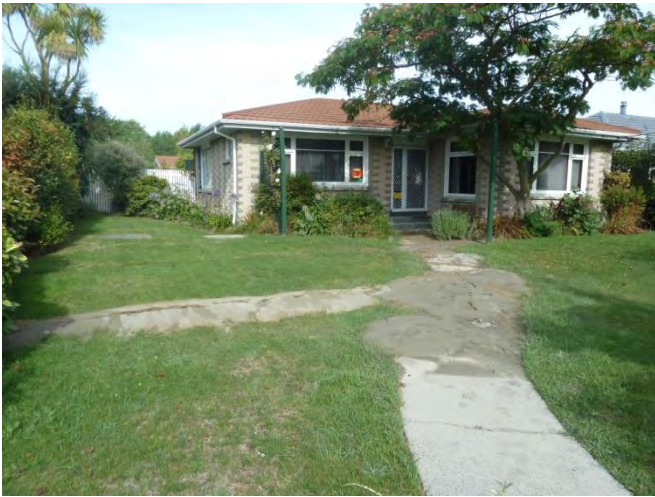
a) Isolated patches of liquefaction ejecta
