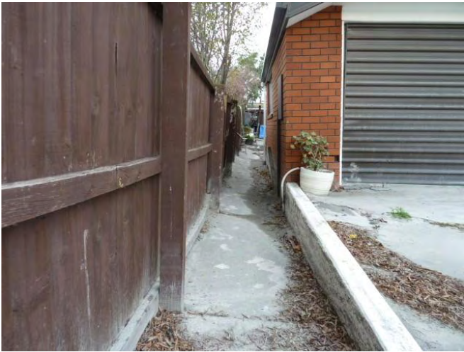
g) Tilting paving slabs as dwelling settled
