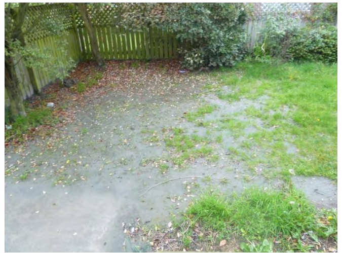
b) Liquefaction ejecta on lawn
