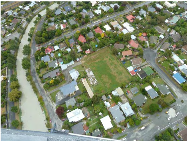
q) Aerial photo of Woolston showing road damage and liquefaction ejecta
