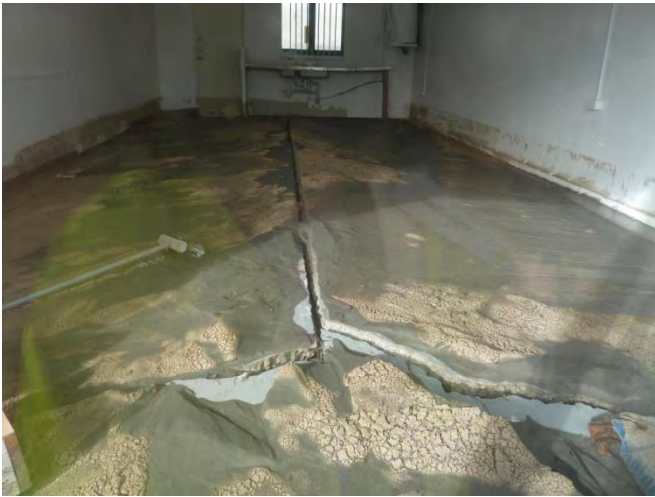
m) Foundation damage
