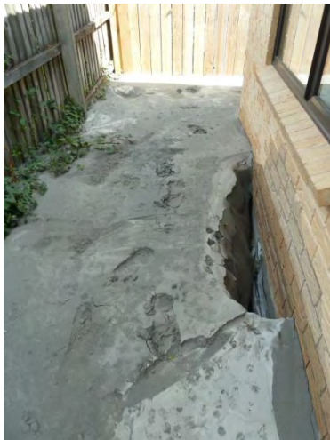
u) Large amounts of liquefaction ejecta
