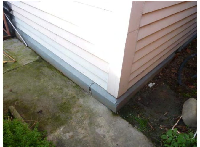
h) Foundation damage
