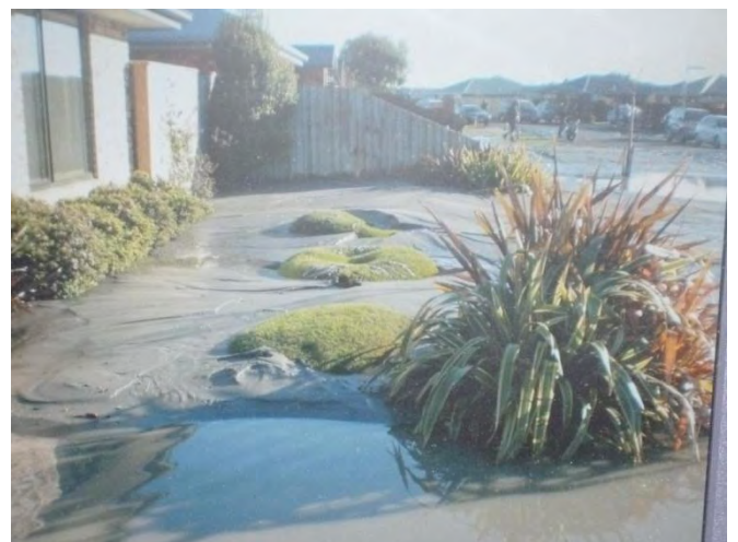
r) Large amounts of liquefaction ejecta
