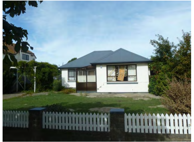
p) Liquefaction ejecta in many areas on lawn
