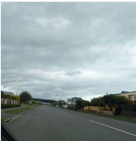
e) View of Aston Drive with little damage
