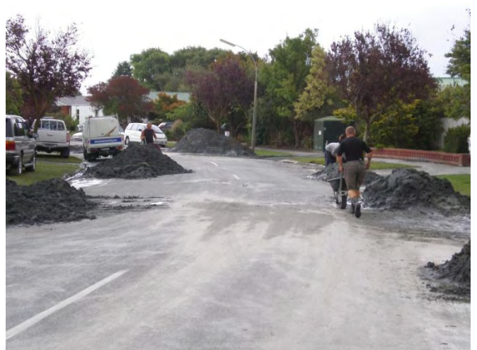
l) Liquefaction ejecta in piles on road
