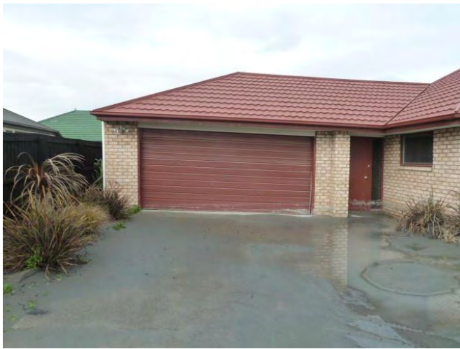
s) Large amounts of liquefaction ejecta and tilting dwelling
