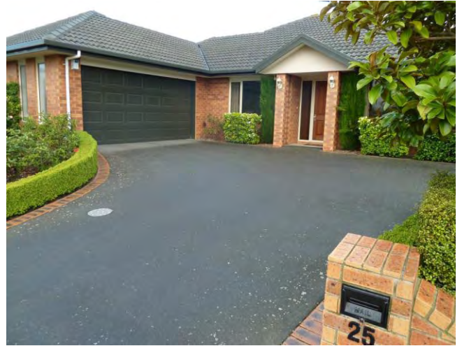
b) Undamaged asphalt driveway
