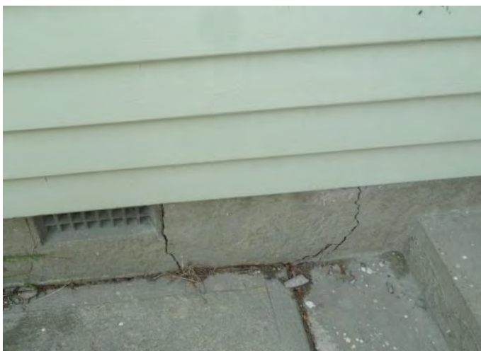
k) Foundation damage
