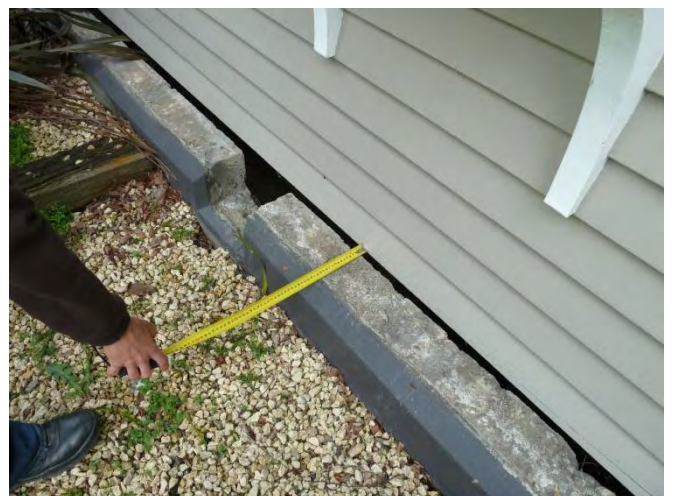
l) Foundation damage
