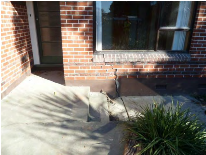
m) Foundation damage
