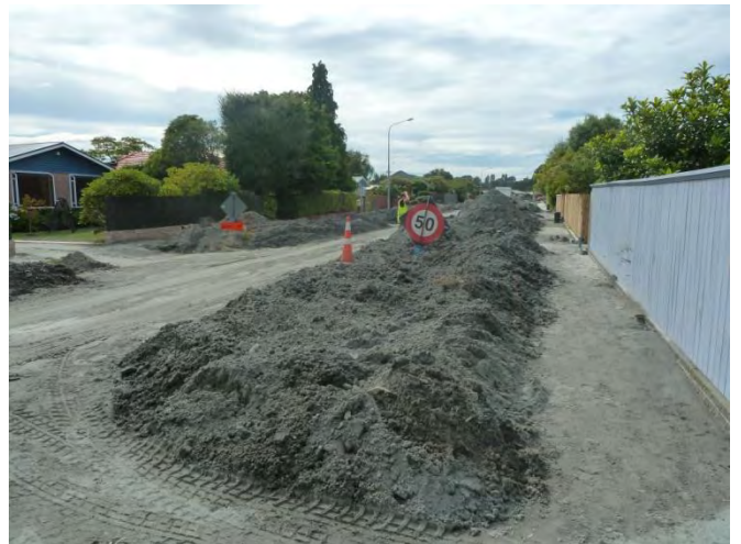
j) Liquefaction ejecta piles along Avonside Drive
