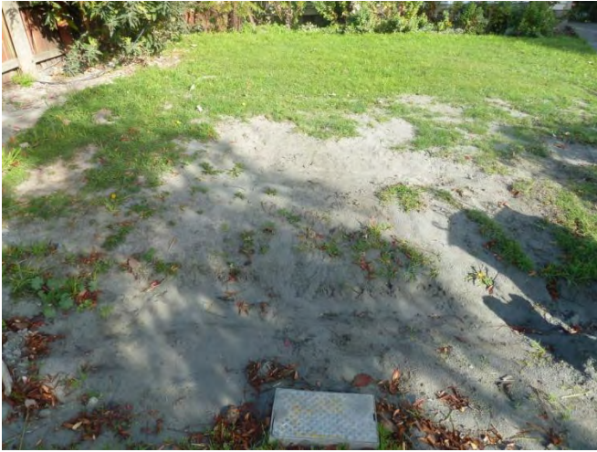
g) Liquefaction ejecta on lawn
