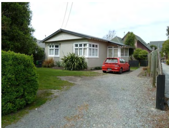
q) Undulating lawns and liquefaction ejecta
