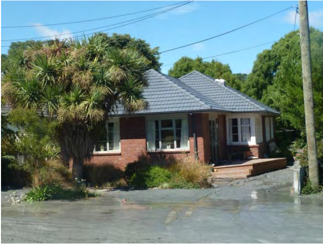
s) Foundation damage, tilting dwelling
