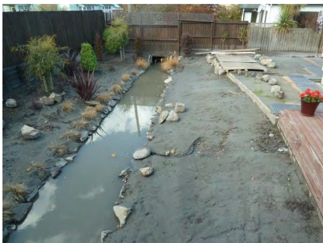
e) Liquefaction ejecta alongside culvert
