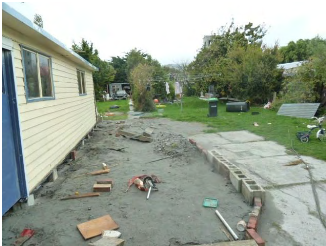
i) Large area of liquefaction ejecta on lawn
