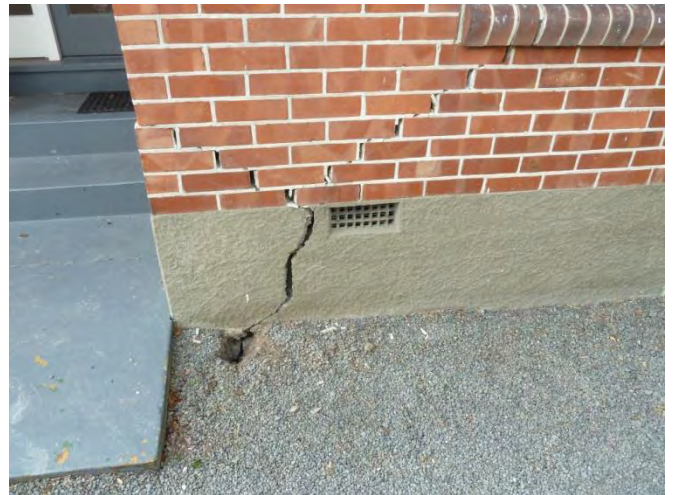
j) Foundation and brickwork damage
